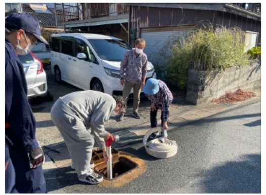
▶茶屋二区消火栓訓練 10/16
